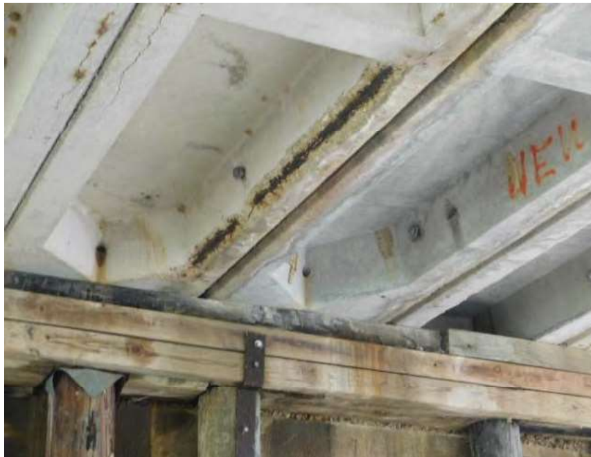
SPAN #3, SLAB "C" SPALLED TO STEEL
