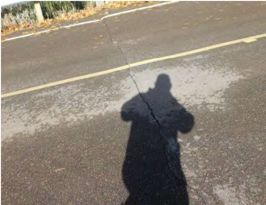
APPROACH #1 ASPHALT SETTLED
