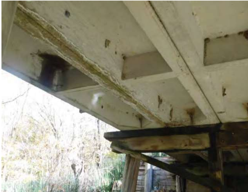
SPAN #2, SLAB "B" CRACKED
