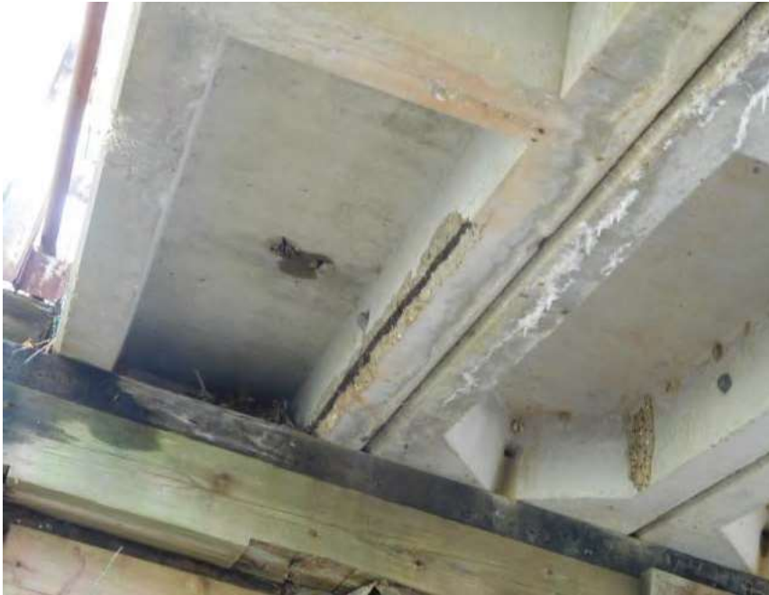
SPAN #3, SLAB "A" SPALLED TO STEEL
